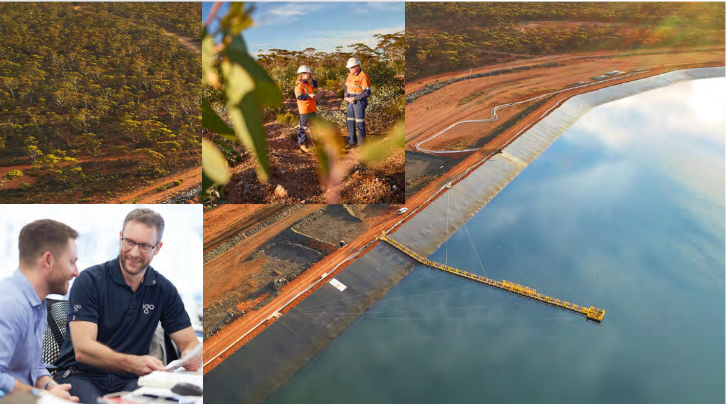
Nova tailings storage facility
