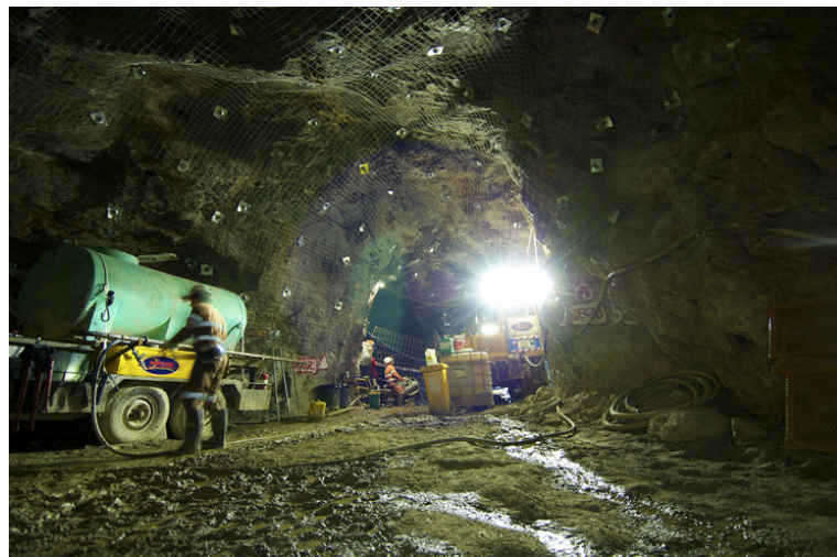
Photo 3: Stockman Project - Underground resource drilling in the Wilga decline.
