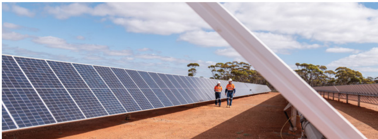
Nova Solar Farm
